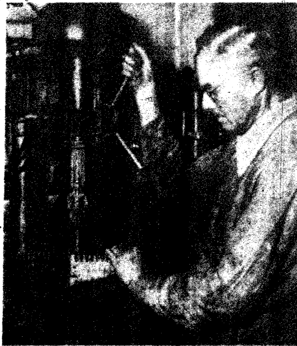
BROTHER Frederick Hensley drills final holes in mould blocks prior to assembly. The trio make their own drills and use a secret process for "cherrying out" or drilling the holes into which the liquid metal is poured. Finished moulds are shipped to many nations.
